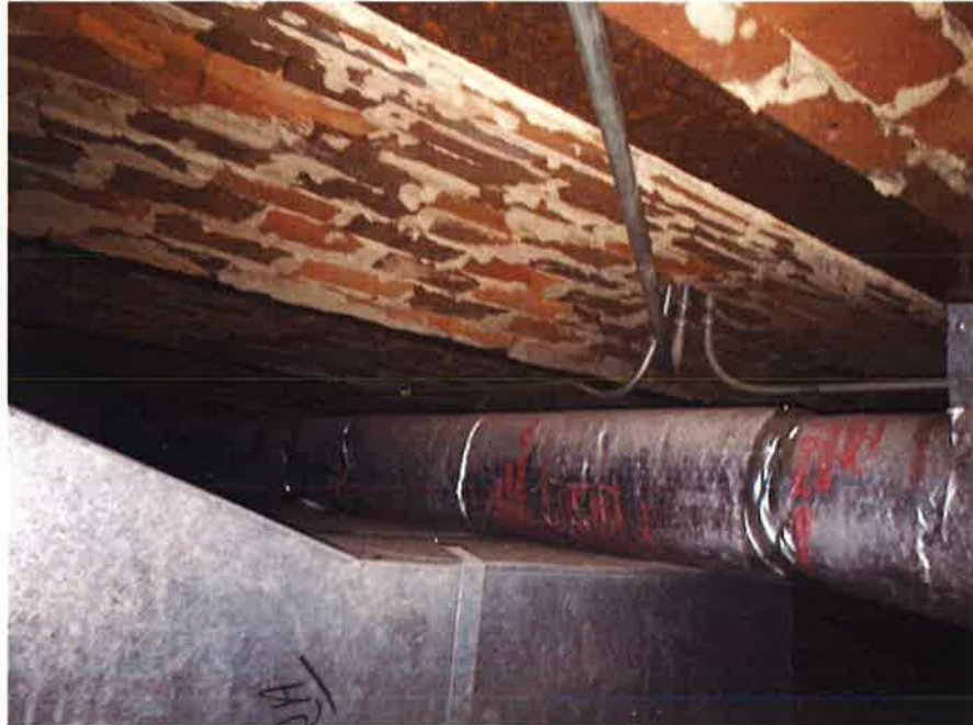
Structural steel and brick floor beneath "secure" room
