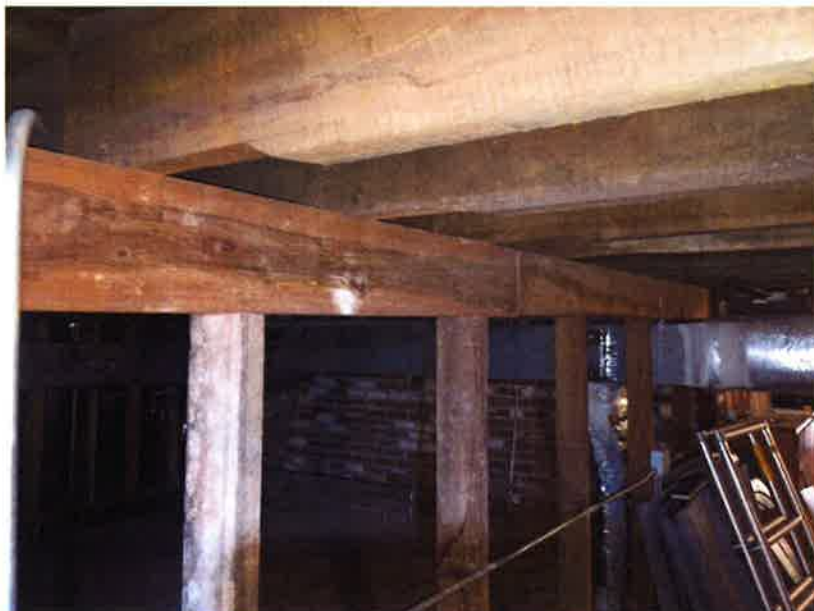
Roof bearing line over steel attic floor beam.
