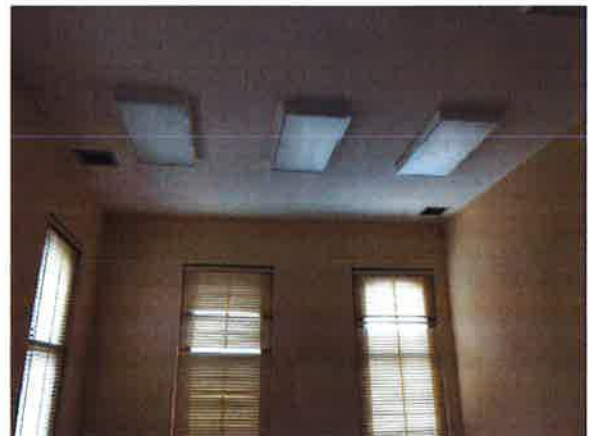
Second Floor – Lighting.
