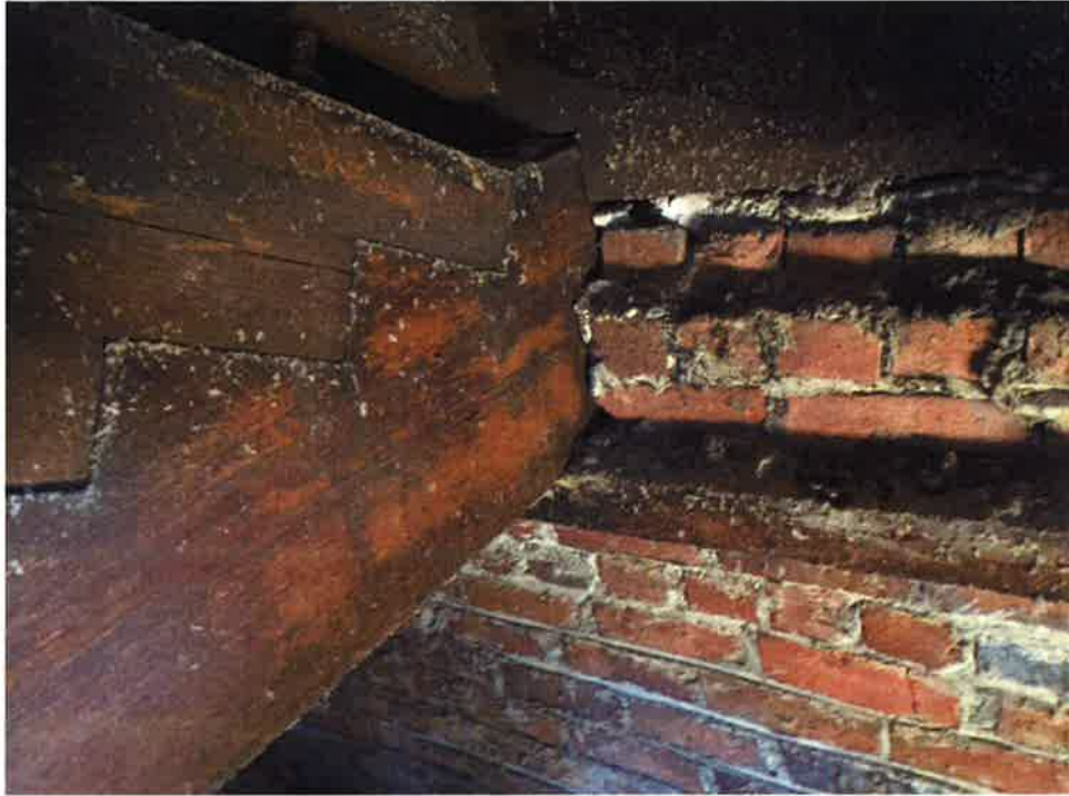
Main truss bearing on north side.
