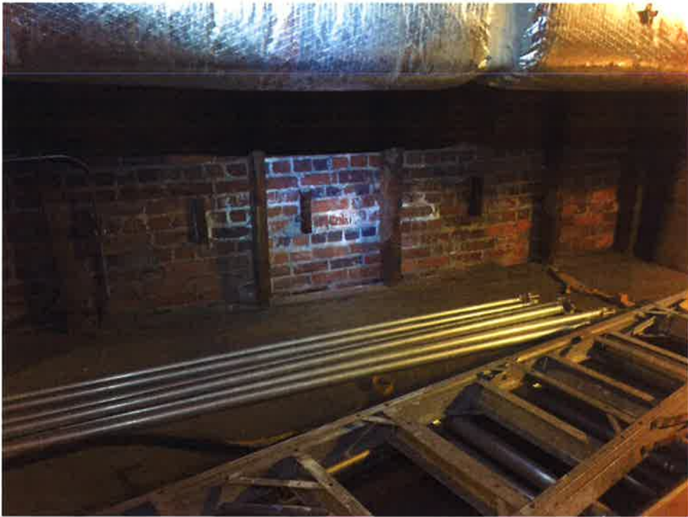
Exterior wall support and outriggers.
