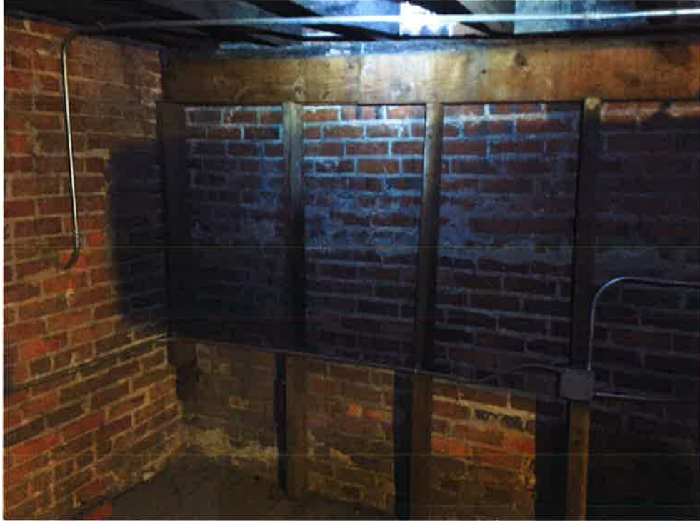
Original roof rafter/joist bearing on exterior wall.
