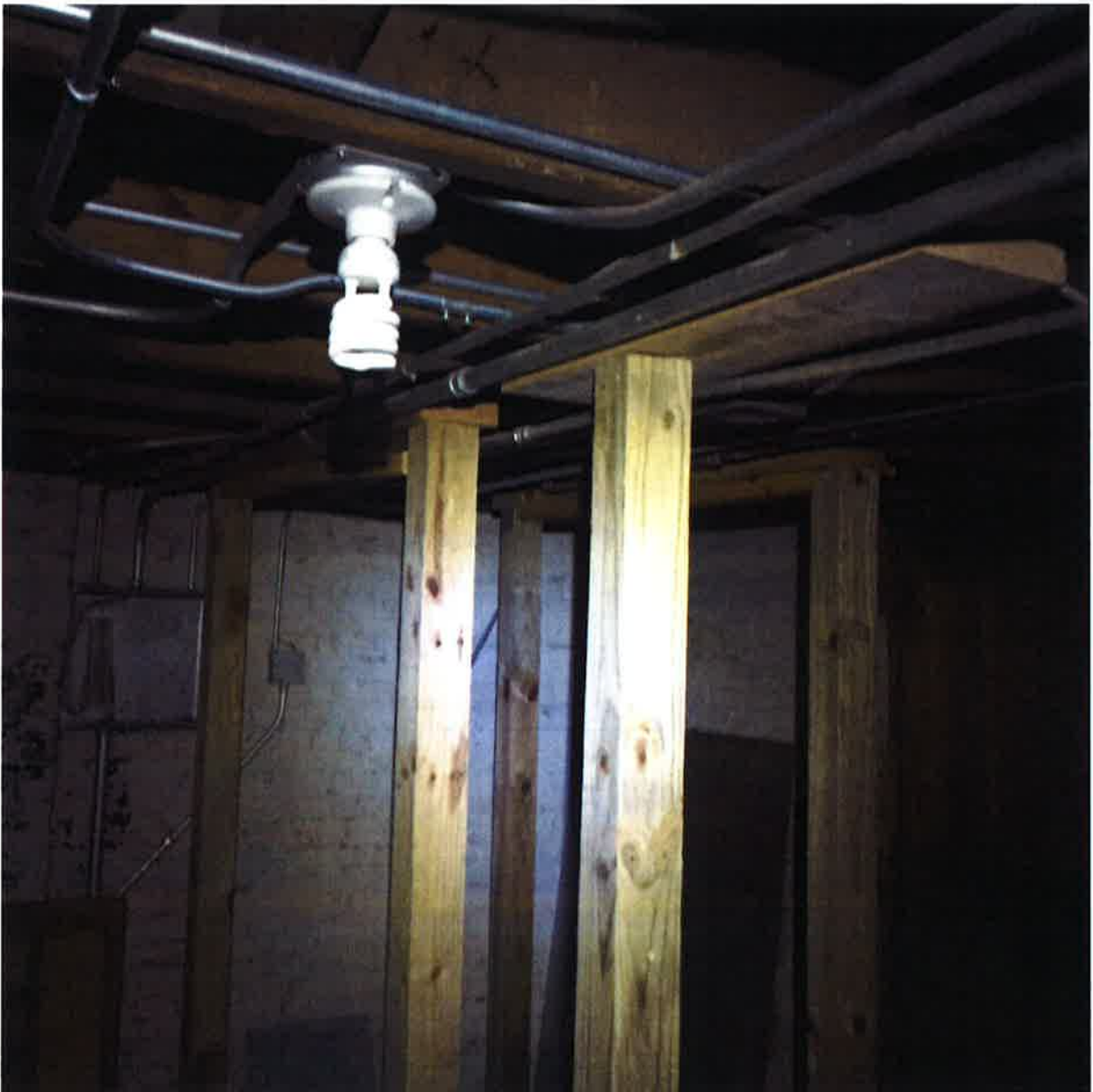
Supplemental framing of roof top units.
