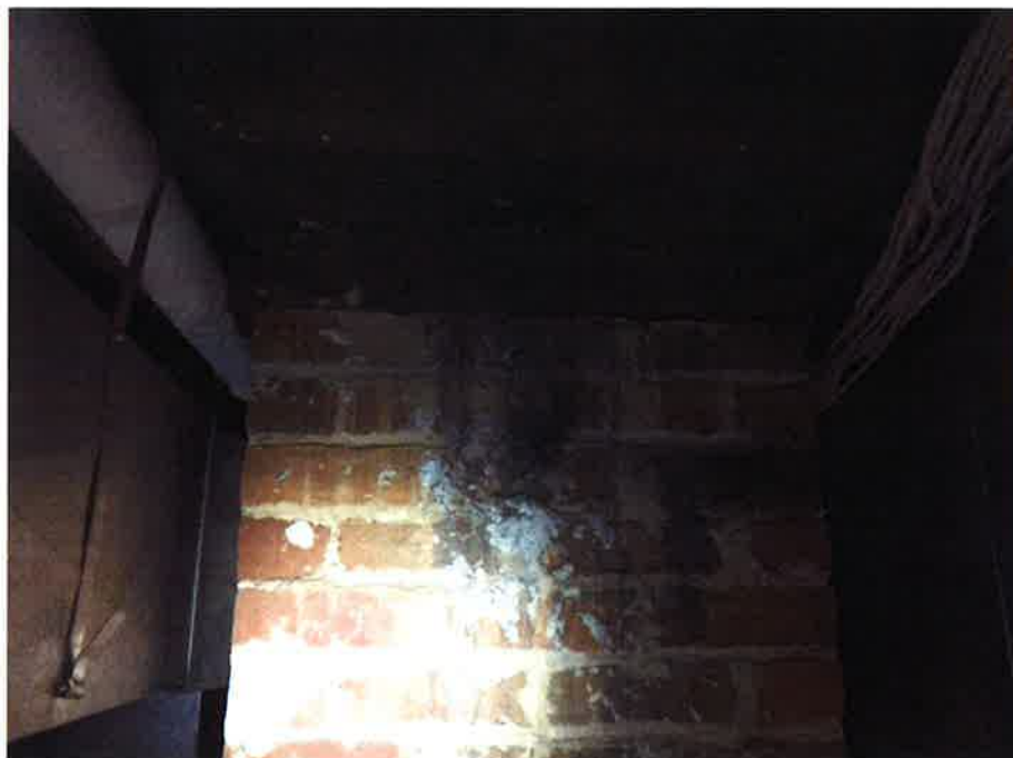
Center pier beneath corridor.
