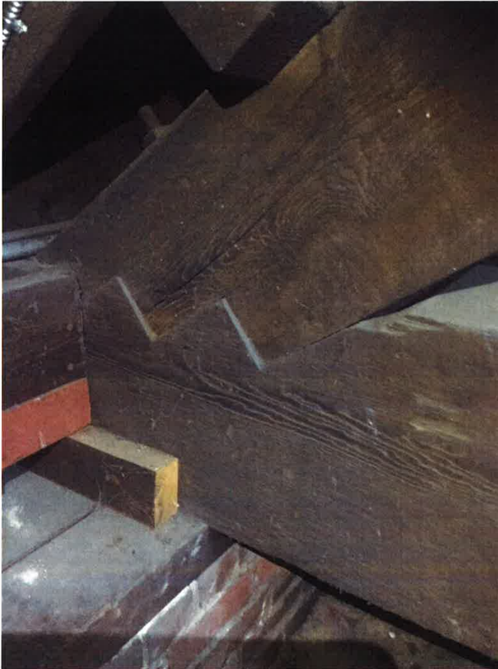
Roof truss bearing. Note notched truss connection with through bolt.
