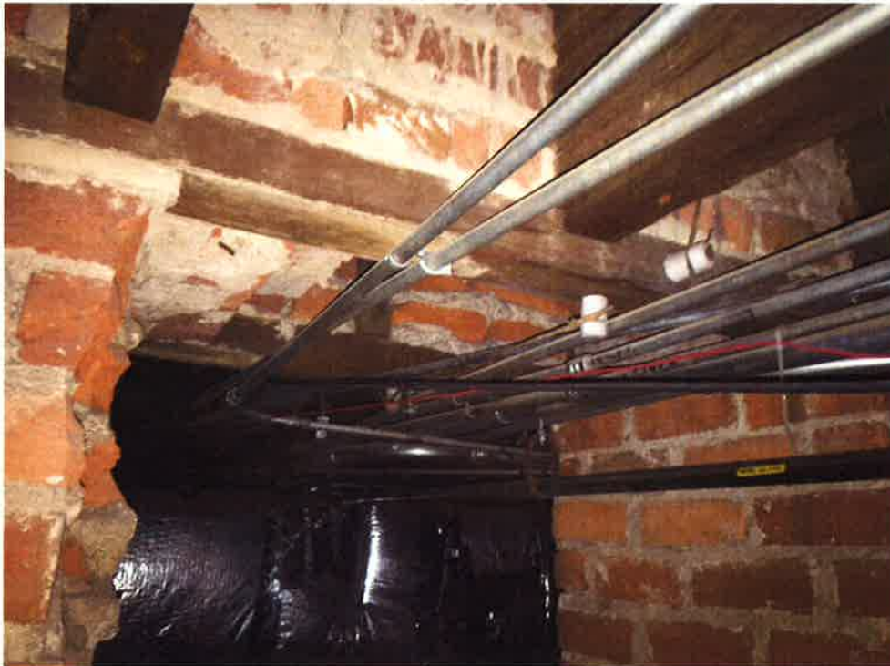
Crawlspace framing and foundation wall at wall penetration
