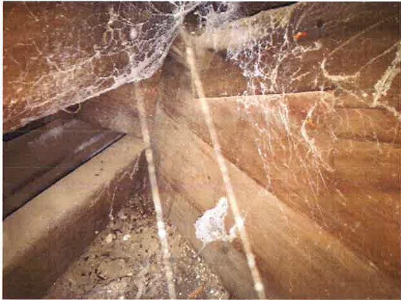
Corner jack truss bearing.
