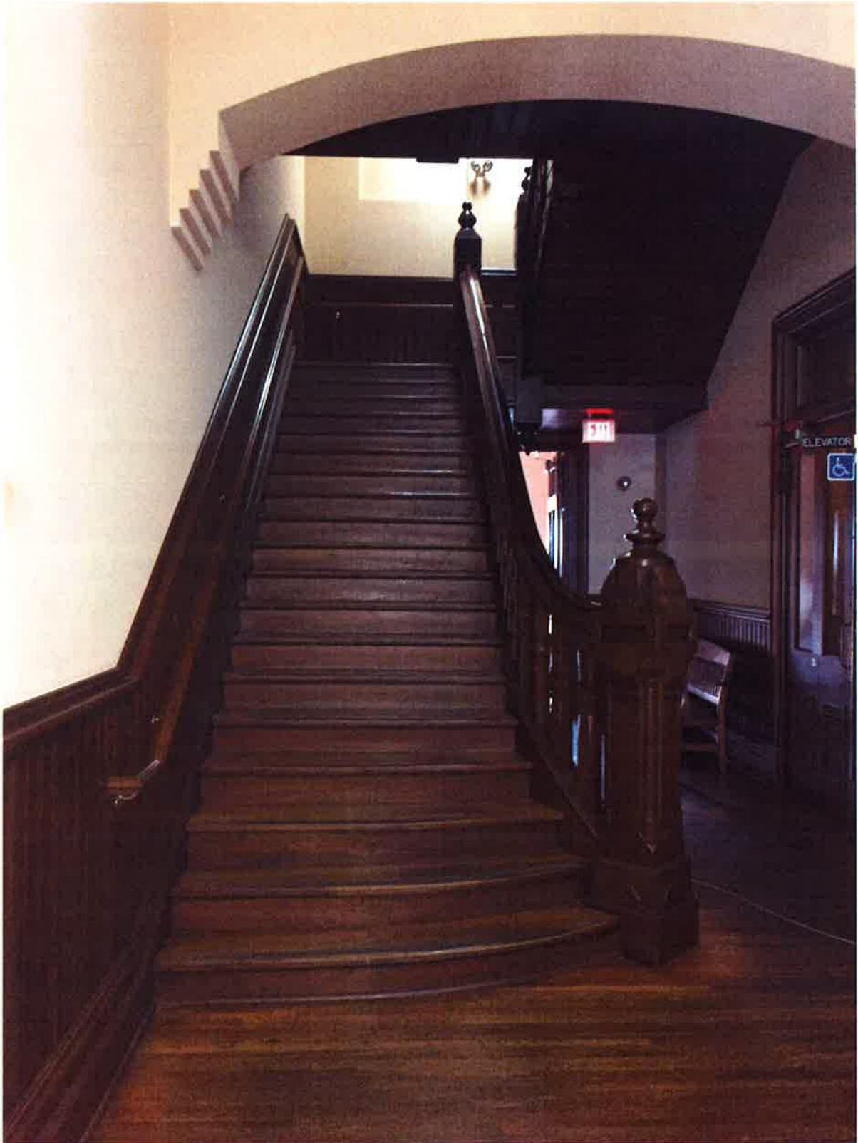
The stair stringers, treads and risers were replaced in 1928.
