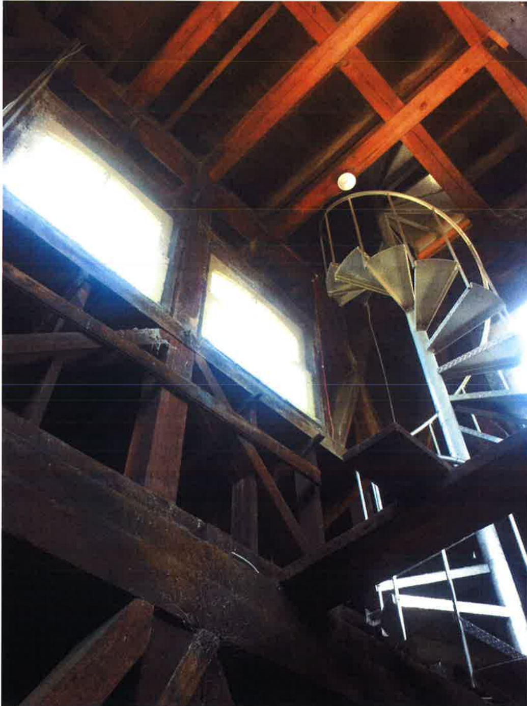
Upward view of clock tower
