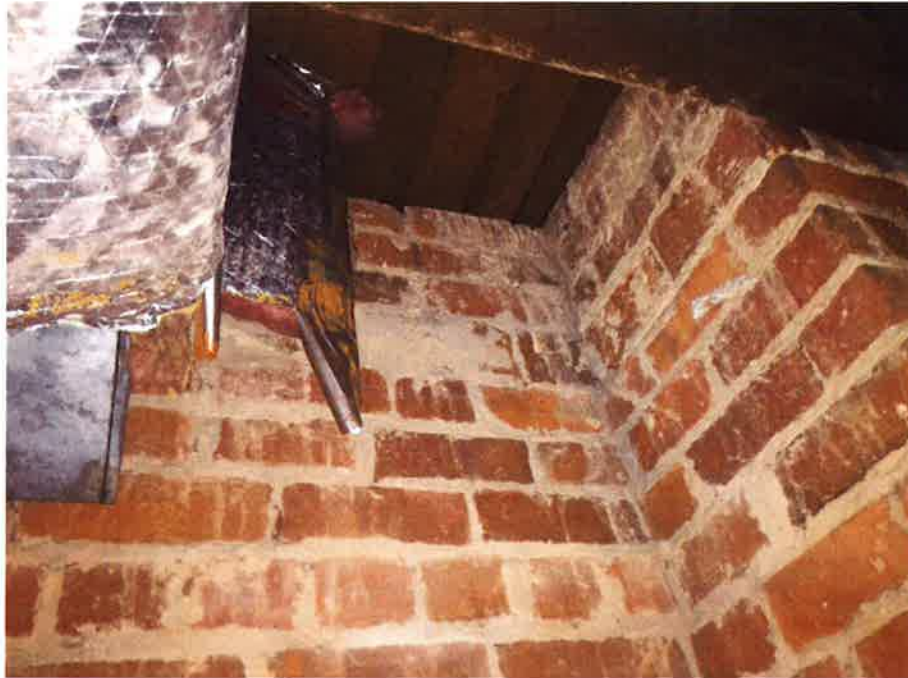
Exterior foundation wall in crawlspace
