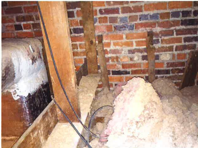
Steel attic floor beam on outer wall of addition.
