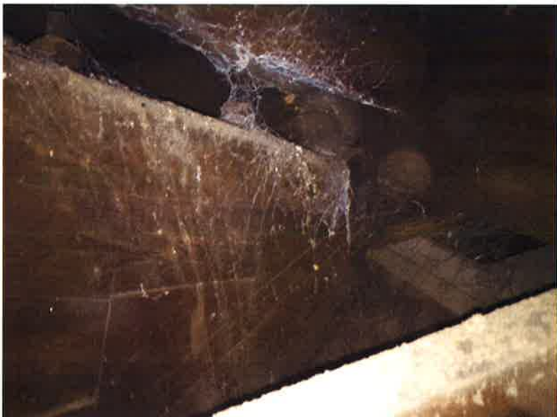
Corner jack truss bearing.
