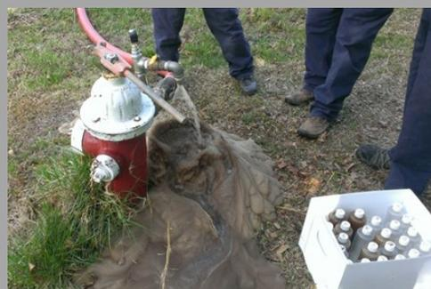
Ice slurry exiting the hydrant
