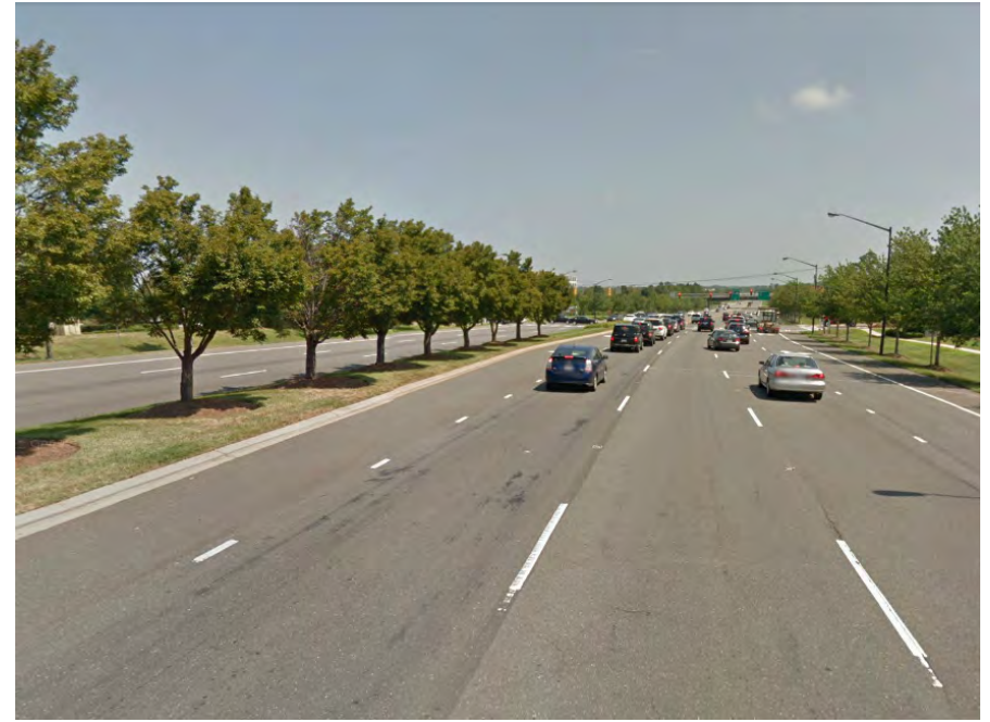
▲ Fig. 4.3 US-521, Johnston Road, Charlotte, NC
