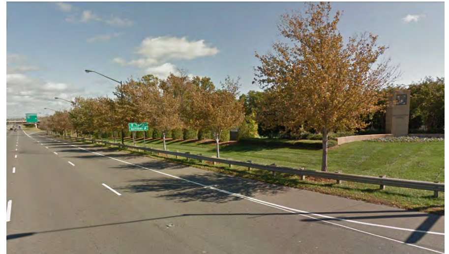
▲ Fig. 10.22 Example of Landscape Creating a Sense of Scale in a 200 ft. Right-of-Way
