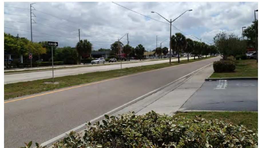
▲ Fig. 4.17 Tyrone Boulevard, St. Petersburg, Florida
