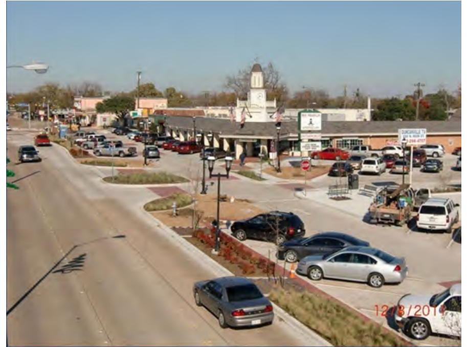
▲ Fig. 6.14 Driveway Consolidation Example, Main Street, Duncanville, Texas
