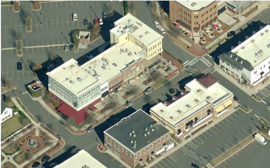
▲ Fig. 9.8 Baxter Village Aerial Photograph
