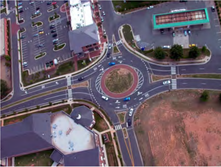
▲ Fig. 5.2 Griffith Street 2-Lane Roundabout, Davidson, NC
