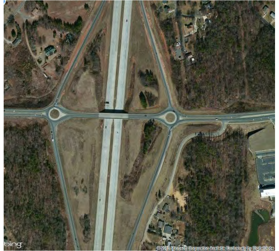
▲ Fig. 5.3 I-485 Moores Chapel Road Exit Single-Lane Roundabouts, Charlotte, NC
