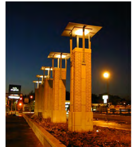
▲ Fig. 10.4 Gateway Illuminated for Visibility at Night
